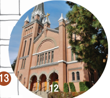
12 St. Thomas Catholic Church 919 E. Indiana Ave. 1909
