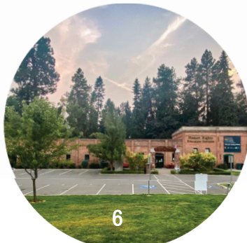
6 Inland Empire Railway Substation 414 W. Fort Grounds Dr. 1904
